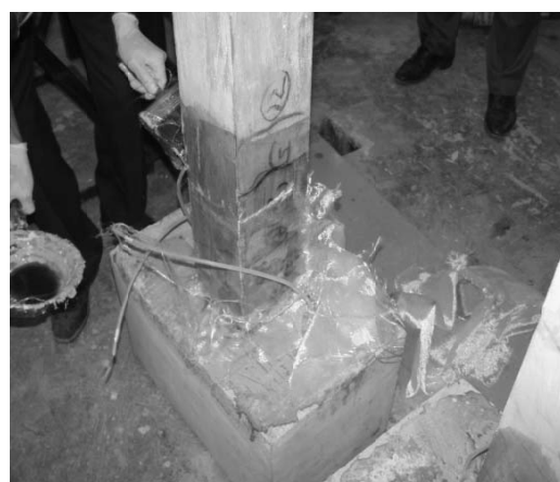
Fig.9 Installation of prefabricated composit sheets
